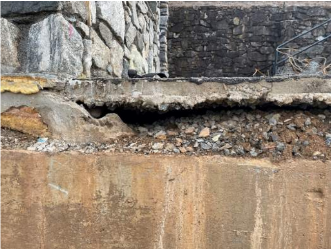
^ Gap below sidewalk – asked H&M to remove portion of walk to explore extents of hole
