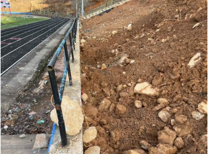
^ Demo at base of grandstand area, looking east
