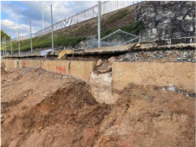
^ Raker beam remnants between retaining wall sections
