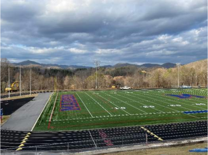
^ Visitor grandstand demolition, across field
