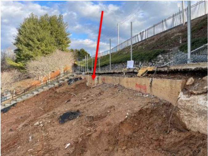
^ Demolition – arrow at undercut footing
