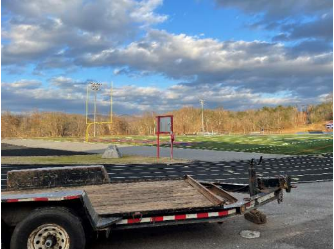
^ Visitor grandstand demolition, across field
